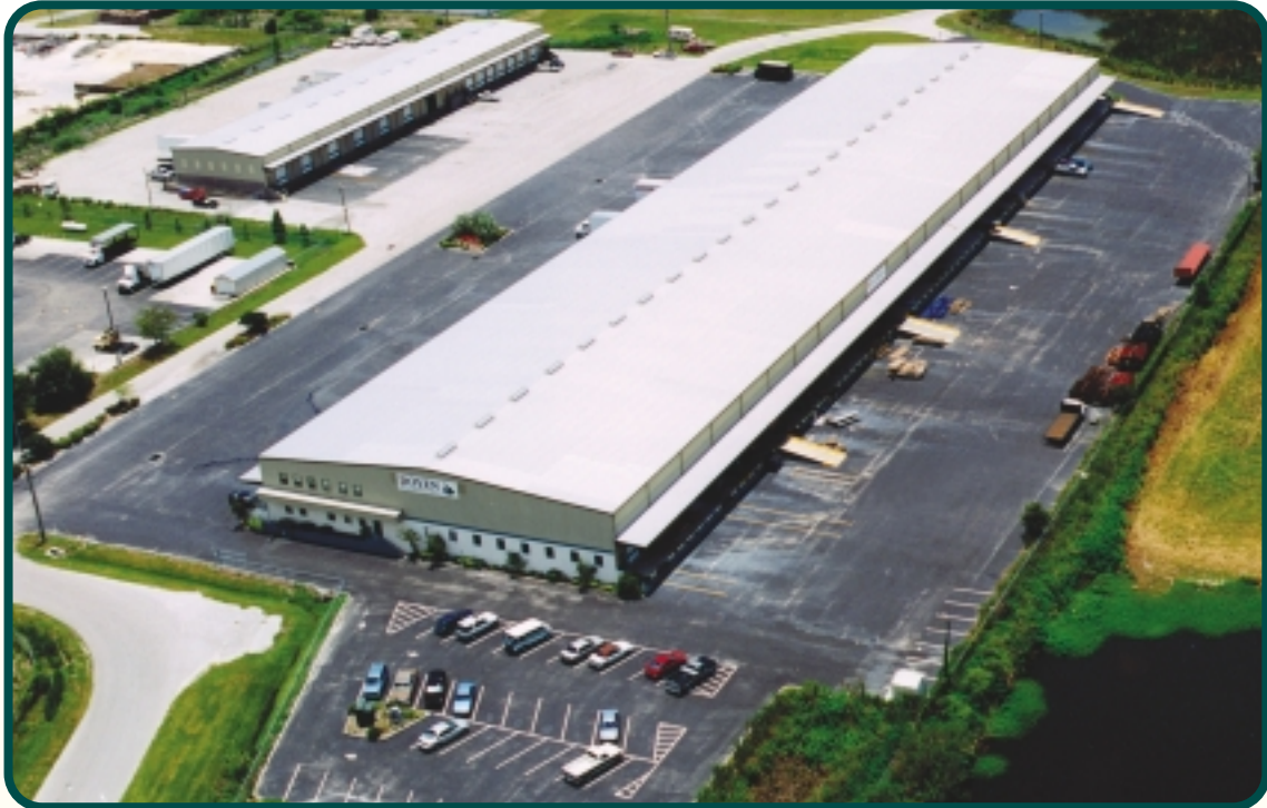
Photo: Aerial Innovations, Inc.
