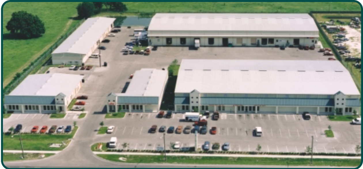
Photo: Aerial Innovations, Inc.
